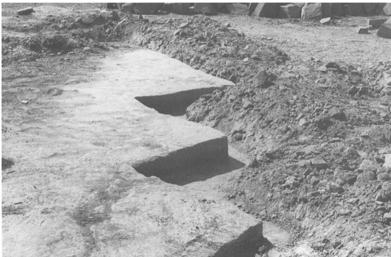
3. Excavation shows where paving has been removed from court.
