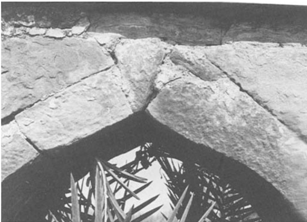
21. Detail. Arch of aqueduct.
