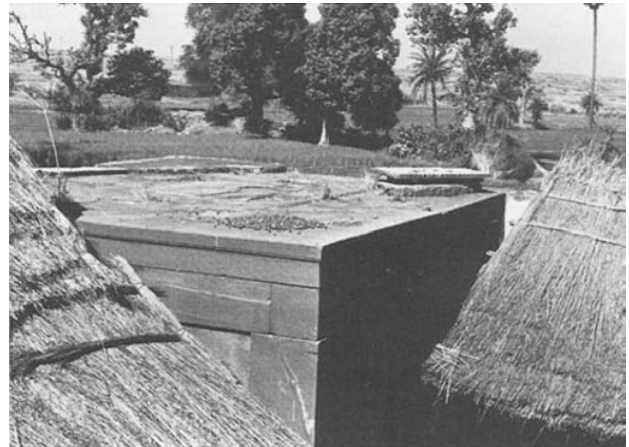
24. Detail. Construction of hammam. Shows densely settled nature of site.
