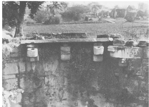
22. Interior of well showing bracket.
