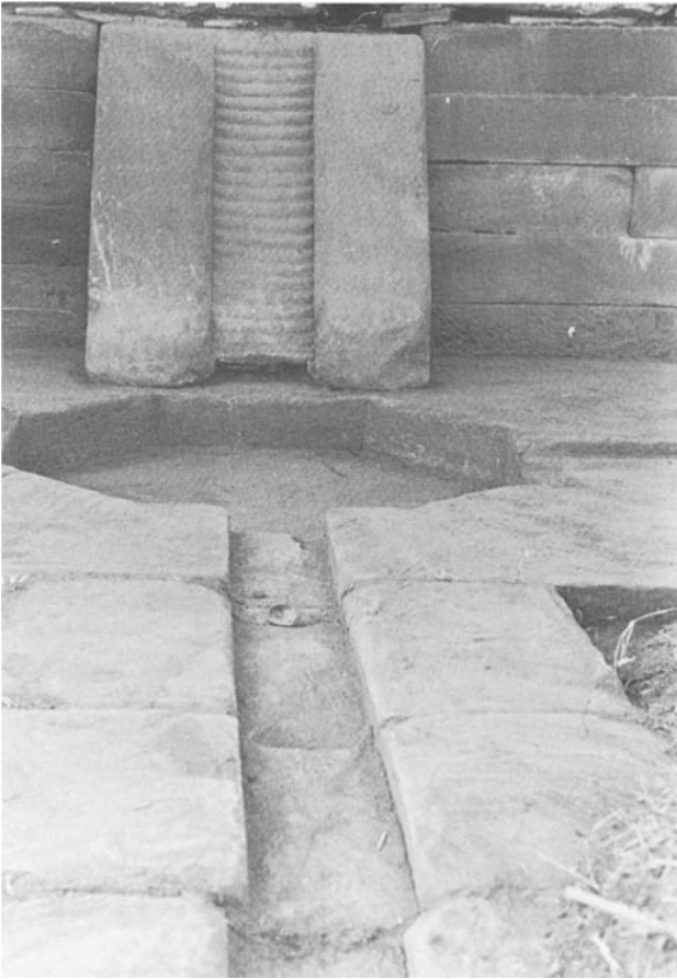
2. Waterchute from Timurid pavilion to rock-cut pool.
