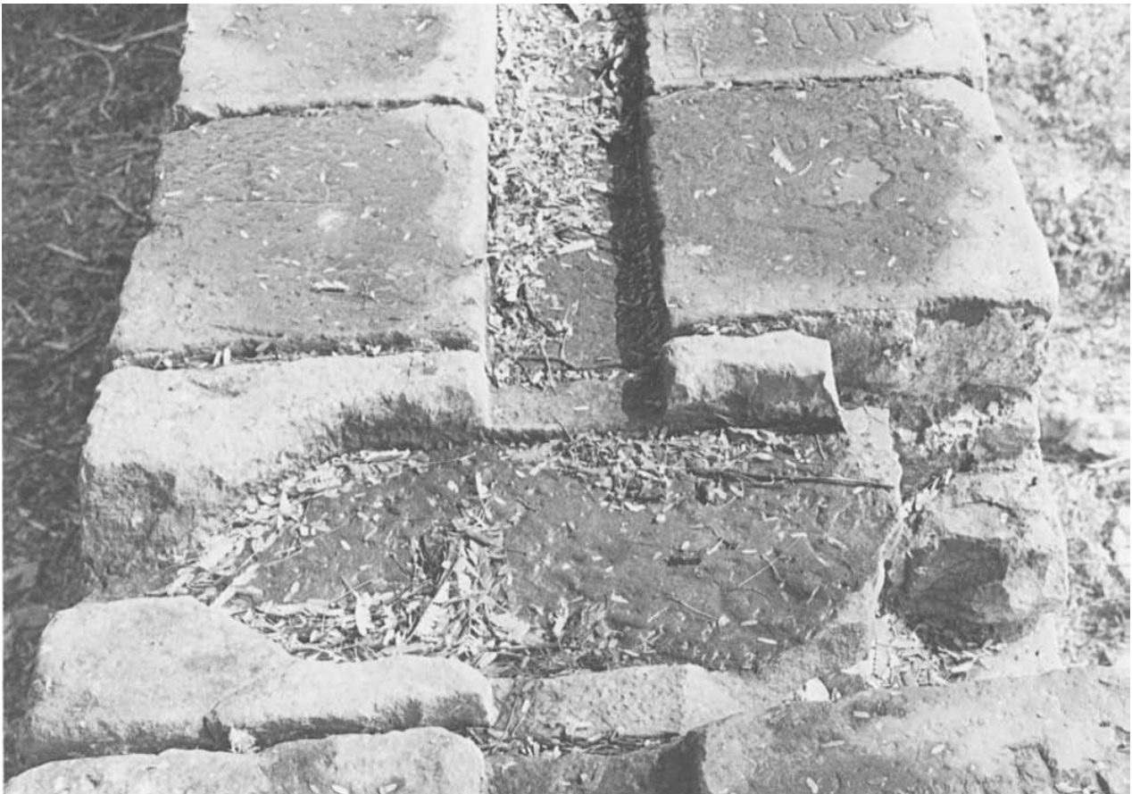
19. Detail. Basin in watercourse on aqueduct.
