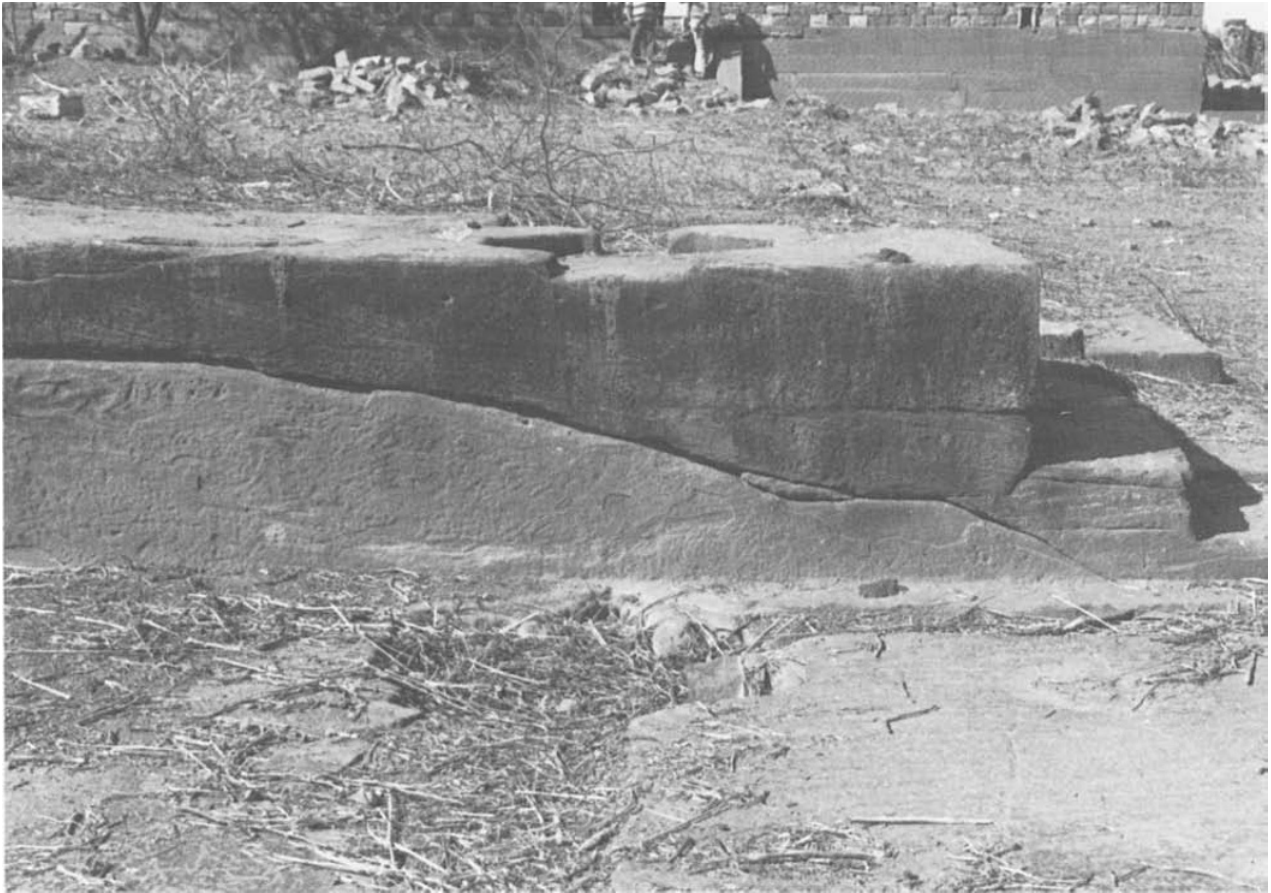
5. West wall of central terrace showing fracture in sandstone.
